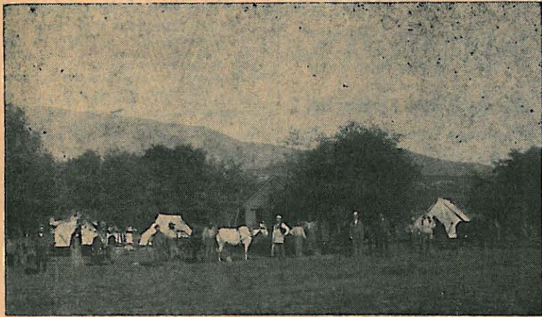
Mr. Arnold and workmen on the site of his large home on the day they gathered to start the foundation. This site is now Dinosaur Land.
