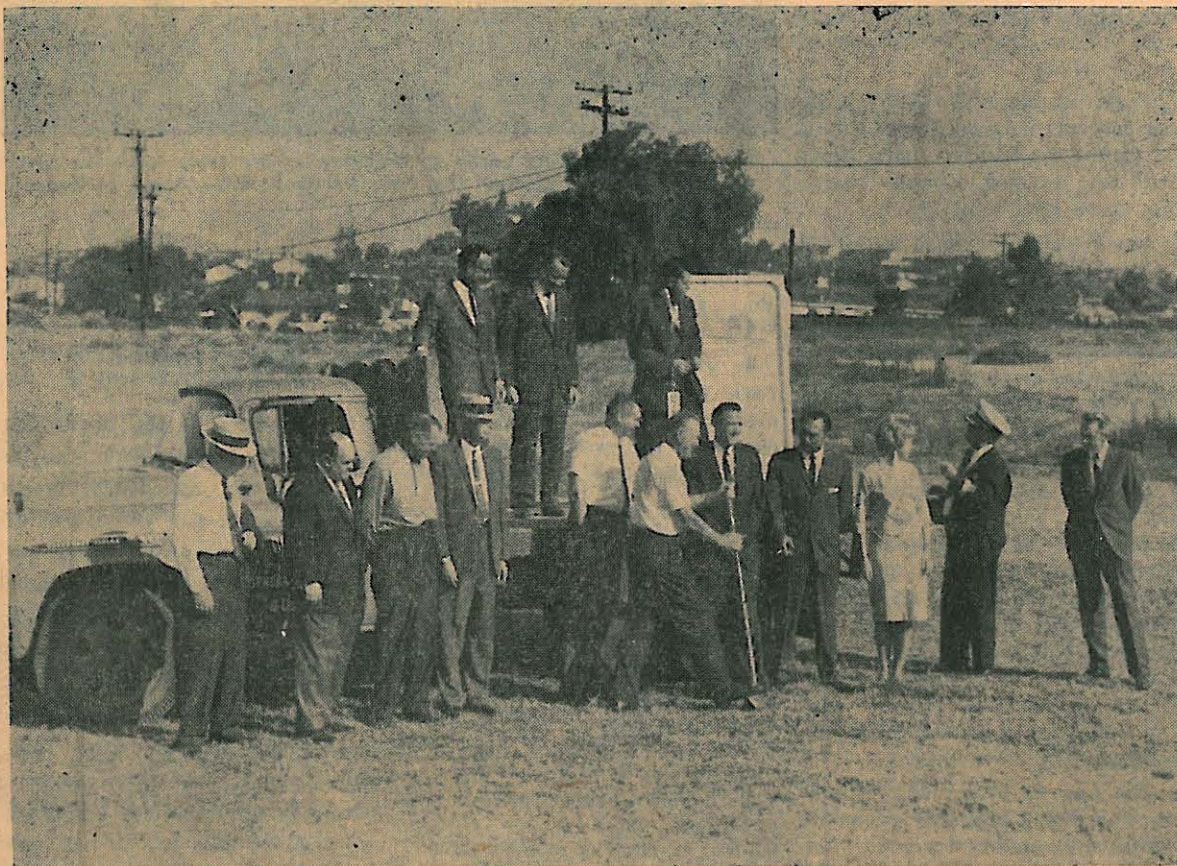
El Cajon Vice-Mayor Lloyd Loftus turns the first shovel of earth at the Ground Breaking Ceremonies for El Cajon Valley Hospital's new Medical Office Building. Bea LaForce Photo
